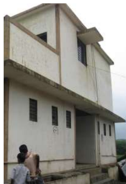
Subsidized Community Toilet Block constructed in the NMMR region of Mumbai.
