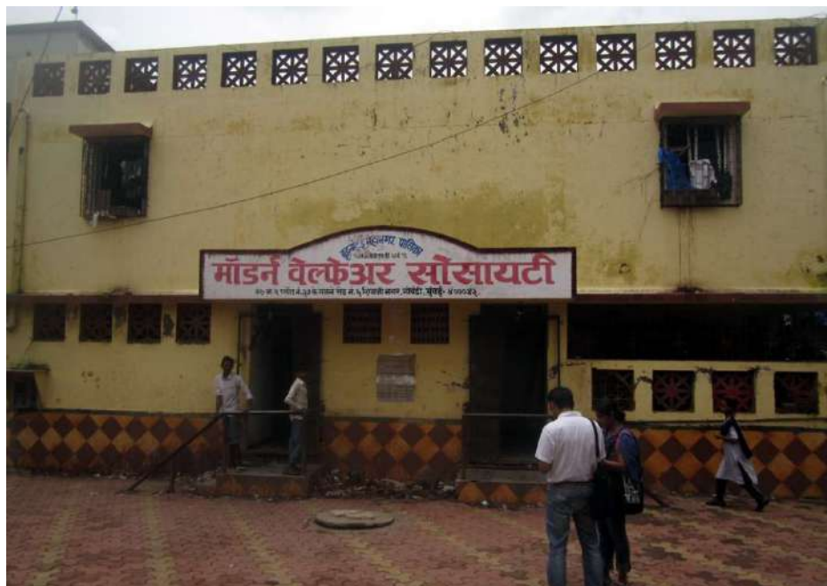
Toilet Block with separate entrances for men and women at Govandi. The caretakers room can be seen at the top.
