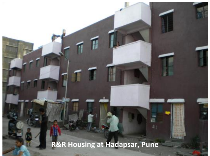
In-situ housing at Dharavi, Mumbai
