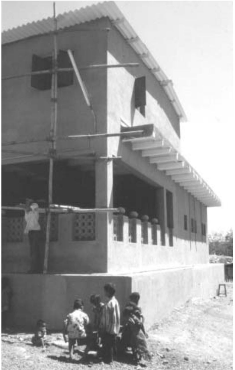
Photo 2: The community-designed Chikhalwadi toilet block in Mumbai under construction. Credit: Homeless International
