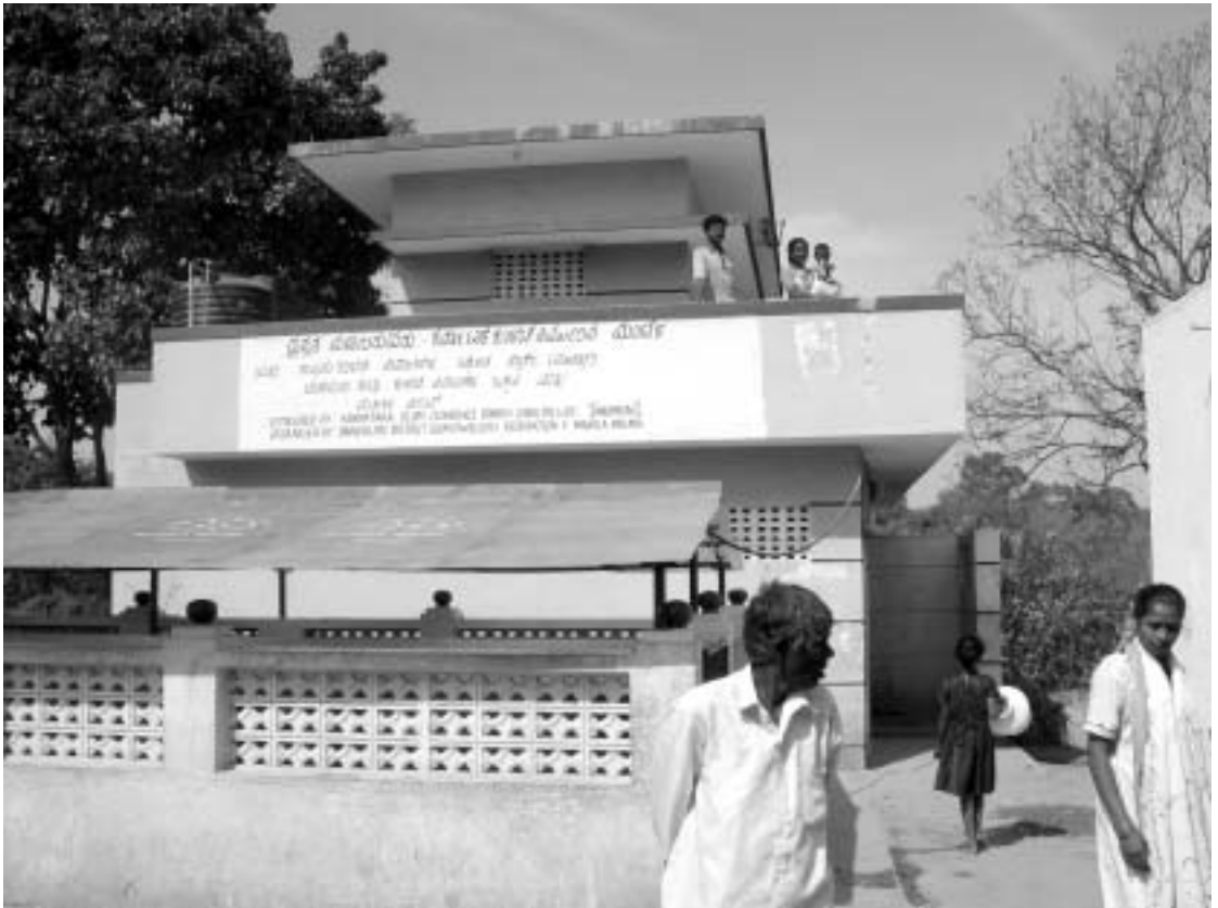
Photo 1: Aundh toilet block built by the community in Bangalore. Credit: Photo provided by the UK charity, Homeless International
