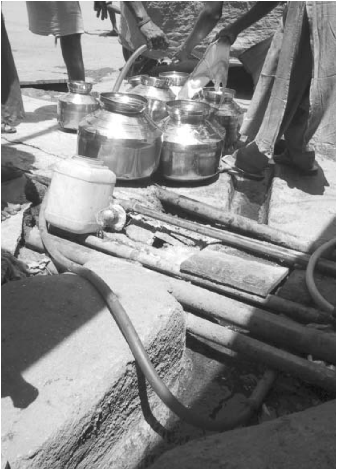
Photo 2: Tapping low-pressure piped water supplies. Credit: SPARC
