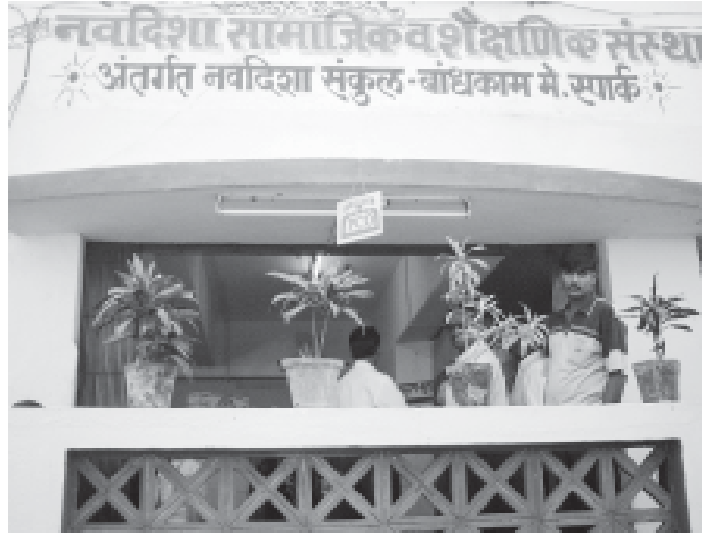
The Navdisha toilet at Govandi is an example to a city as far away as Tirupur in Tamil Nadu.
